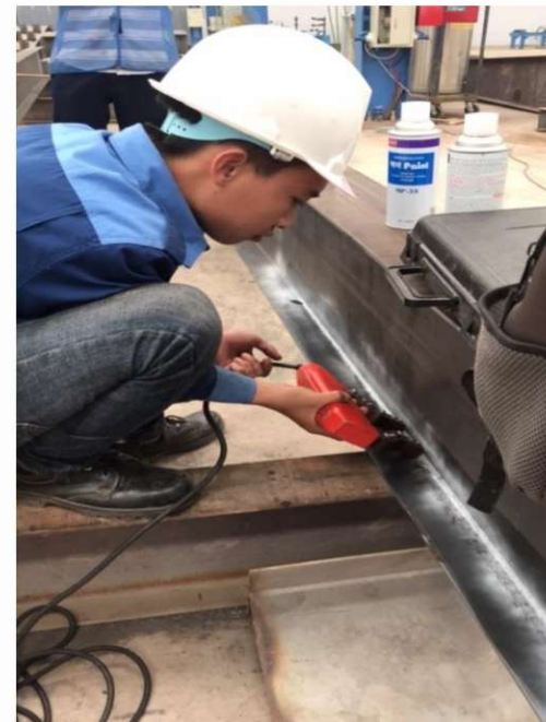
Checking auto welding line by magnetic
